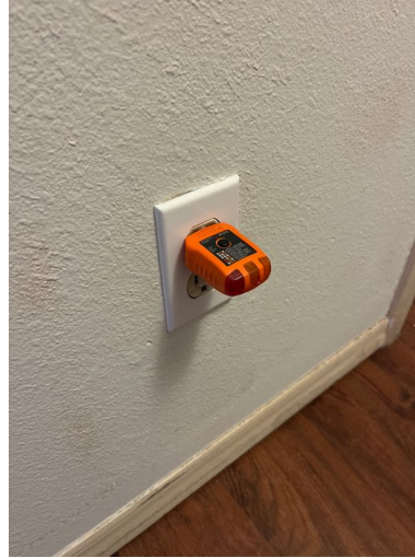
Unit A Hallway
