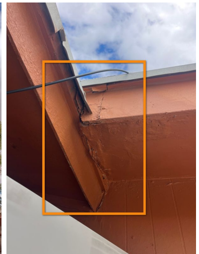
Rear of Structure
