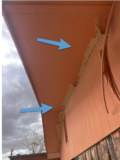
Rear of Structure
