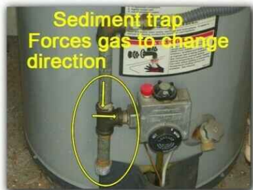
Example of properly installed sediment trap.
