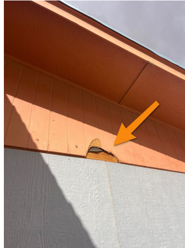
Rear of Structure
