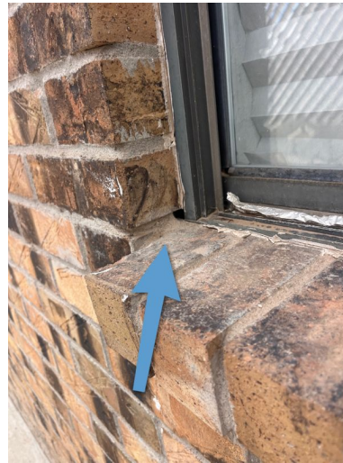
Left Side of Structure
