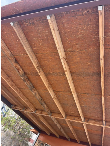
Rear of Structure
