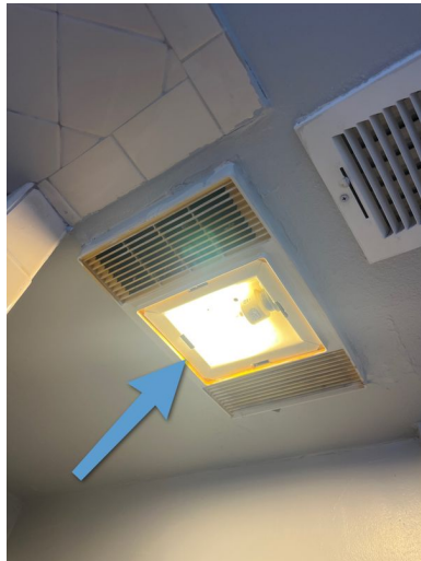
Unit B Hall Bathroom
