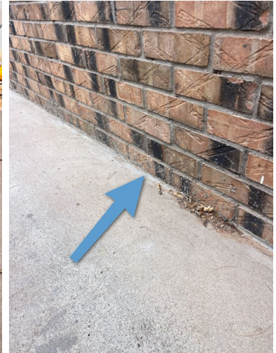
Left Side of Structure
