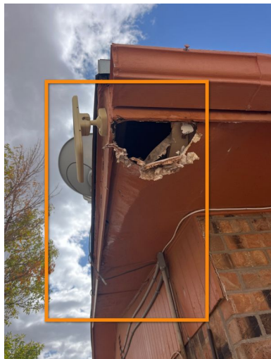
Left Side of Structure
