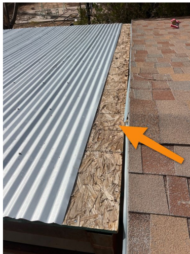
Rear of Structure
