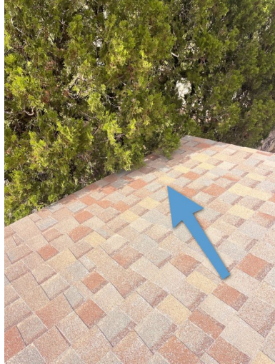
Right Side of Structure
