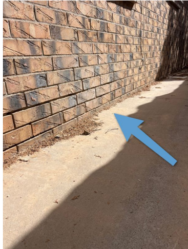
Right Side of Structure
