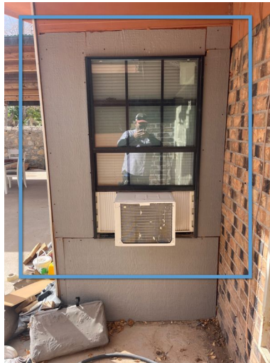
Rear of Structure
