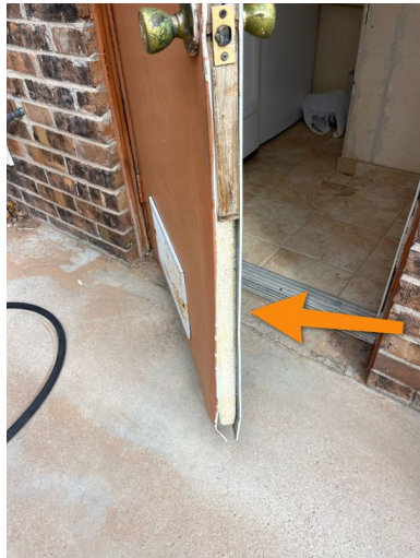
Rear of Structure
