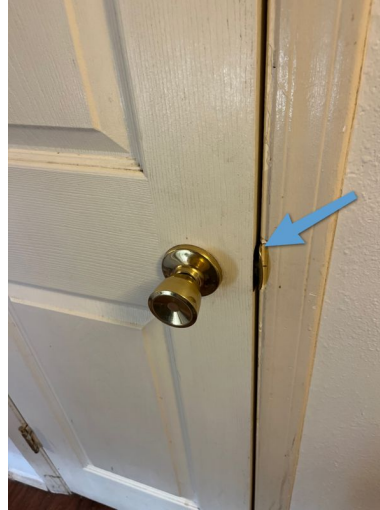
Unit A Hallway
