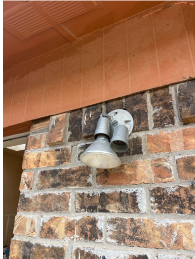
Rear of Structure
