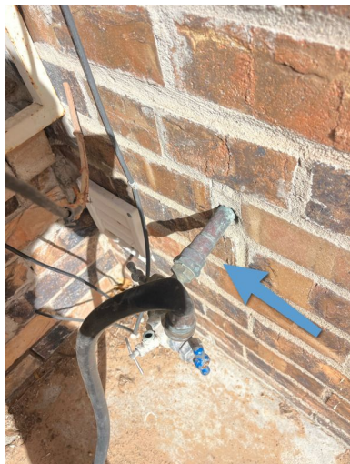
Rear of Structure
