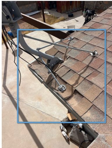
Rear of Structure
