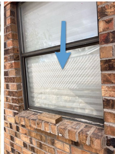
Left Side of Structure
