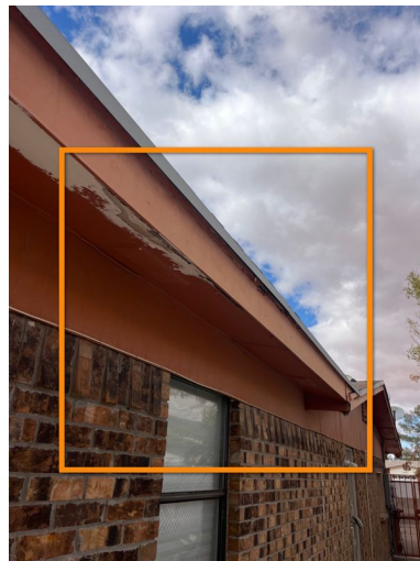
Left Side of Structure
