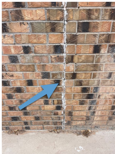
Left Side of Structure
