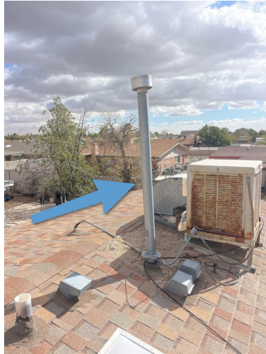
Rear of Structure
