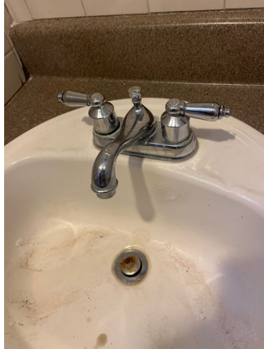
Unit B Hall Bathroom
