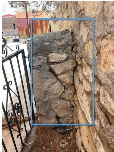
Right Side of Structure
