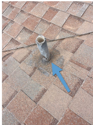
Rear of Structure
