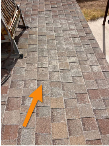
Rear of Structure
