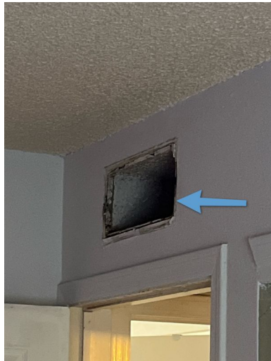
Unit A Spare Bedroom Rear
