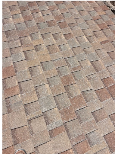
Right Side of Structure
