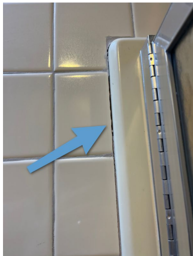
Unit B Hall Bathroom
