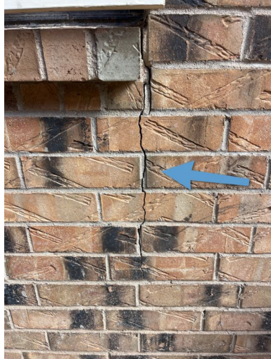
Right Side of Structure
