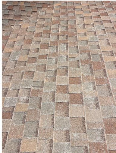
Rear of Structure
