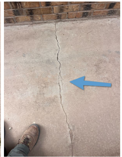
Left Side of Structure
