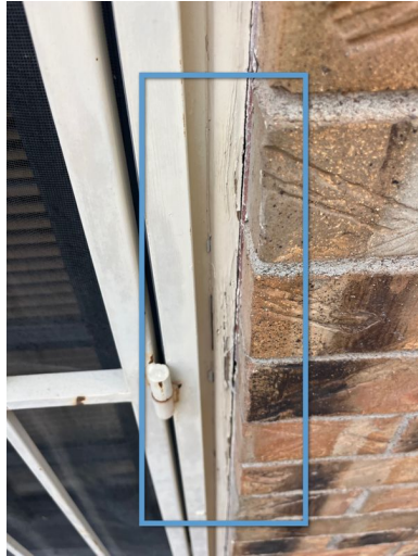
Left Side of Structure
