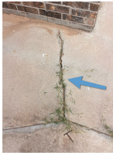
Rear of Structure
