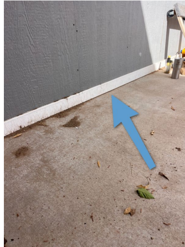
Rear of Structure
