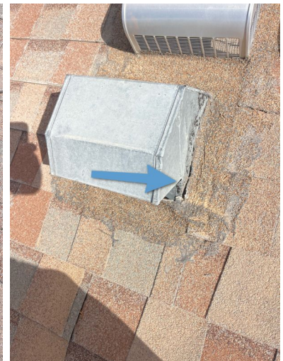
Right Side of Structure
