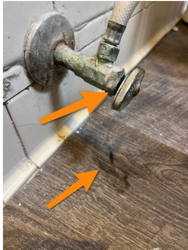
Unit B Hall Bathroom
