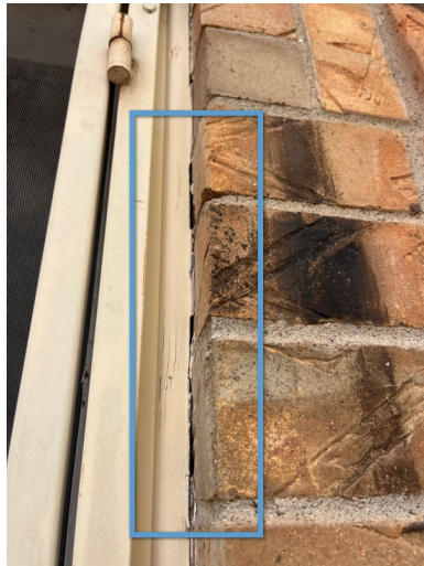
Left Side of Structure
