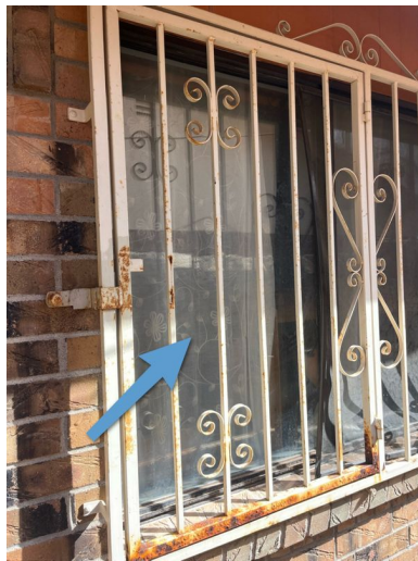
Right Side of Structure
