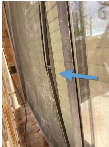
Rear of Structure
