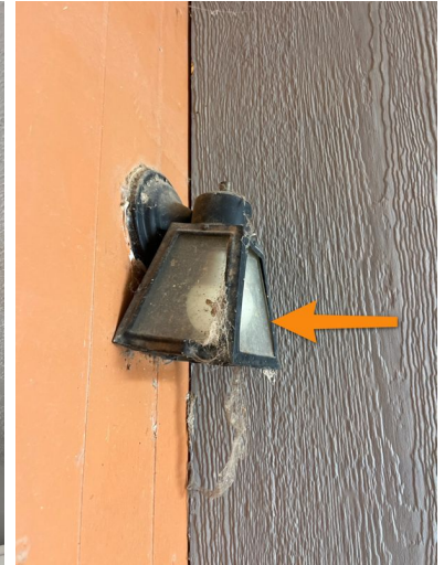
Rear of Structure
